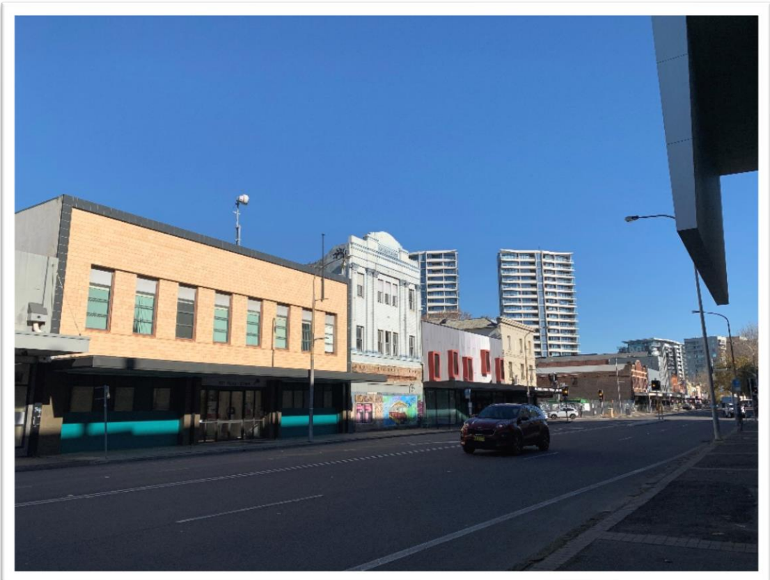
Figure 5: View looking south west toward the building frontage
