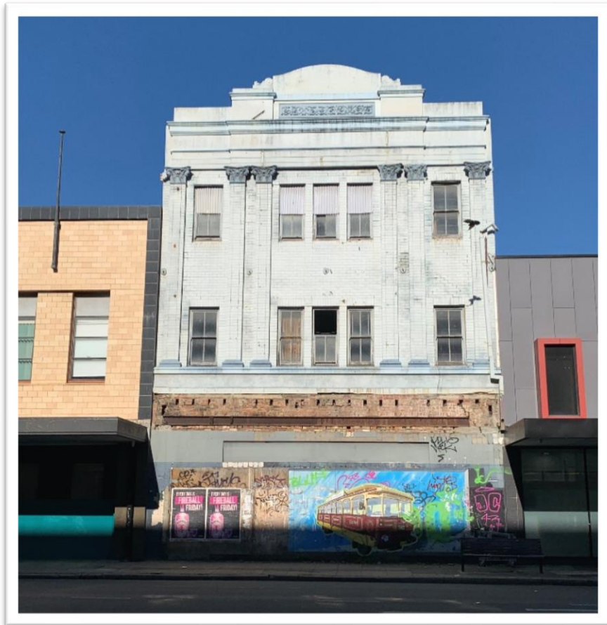
Figure 2: View from Hunter Street looking south towards the building frontage
